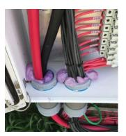
Polywater AFT can be used to seal more than conduits, including solar inverters, riser poles, U-Guards, raceway entrances, and more.
